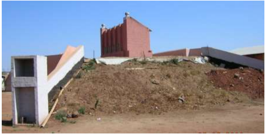
(Fig. 10); South east view of the community hall.
