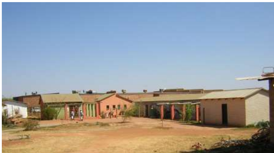
(Fig. 3); The Eco-village “business quarter”; half completed.
